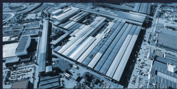
Vicenza plant, ITALY (Total surface: 294.608 m 2 )
